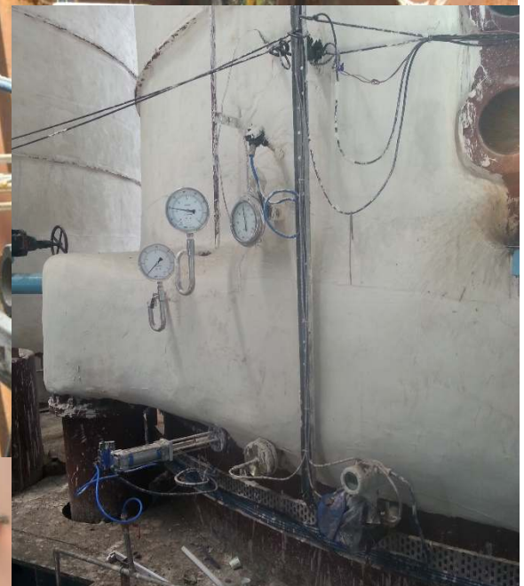
Auto Retracting Self Cleaning Brix Sensor installed on Batch Type Vacuum Pan
